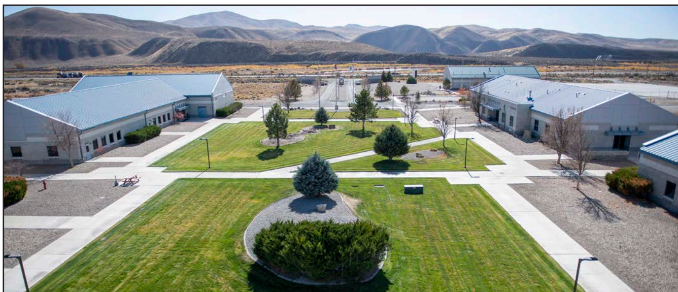
The Elko County Readiness Center, formerly the University of Nevada, Reno Fire Science Academy, sits in the foreground just north of Interstate 80 in Carlin, Nevada. The readiness center is the site of the Battle Born Youth ChalleNGe Academy, set to open with classes in June 2021.
